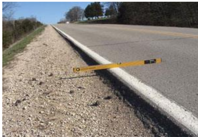
Figure 2. 1 Typical Example of Pavement Edge Drop-Off. Source: Hallmark et al. (2006)
